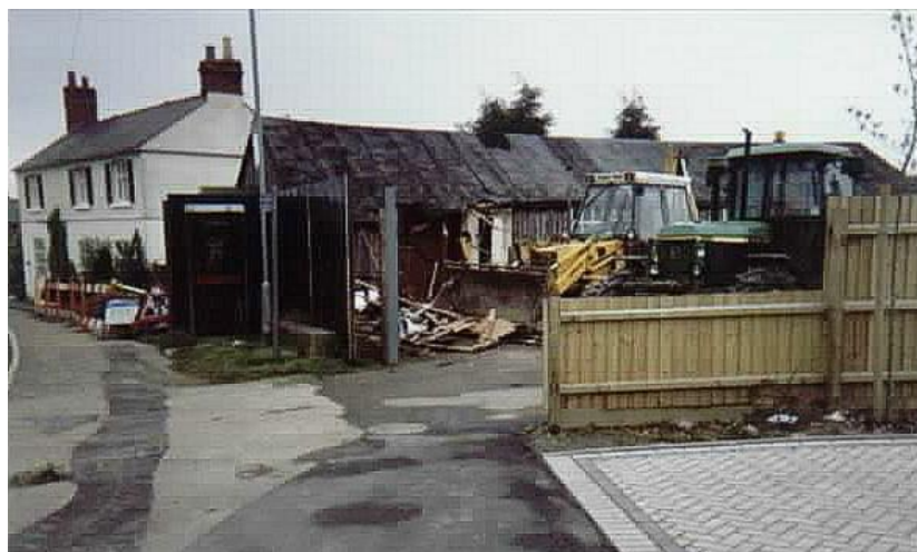
The old hall being demolished in 1993.
